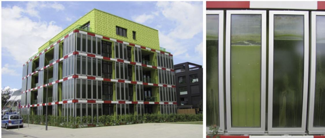
Figure 4 MA-BRF in BIQ house, Hamburg Germany, zoomed image of PBR panels being used as façade (Boloria and Thakkar, 2020).
