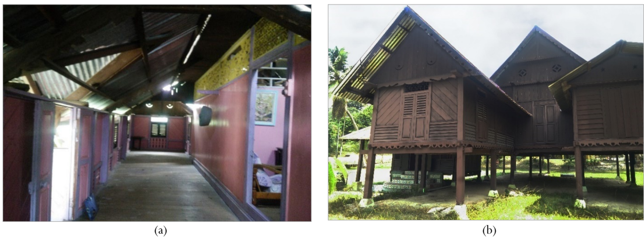
Figure 5 Plenty of full-length operable windows at the body level, ventilated kepala tangkap , pagar musang and lubang angin (a), and the ventilated gables end and full-length wooden panel operable windows with louvers paneling (b)
