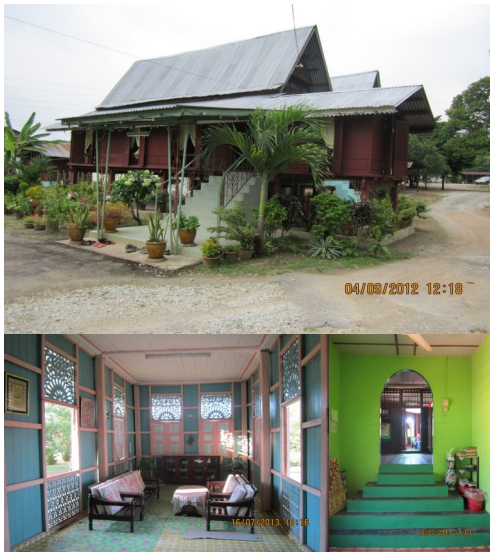
Figure 6: The geometry of high pitched roof, on-stilts structure, quality of materials, surface, craftsmanship and spatial segmentation of frontal and posterior zones contribute to the high level of values in the originality of Malay traditional house design.
