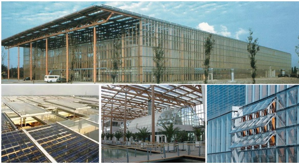
Figure 3: Mont Cenis Training Center, Herne-Sodingen, Germany
