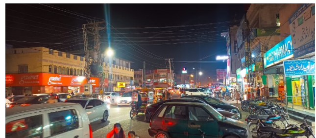
Figure 16A. Extensive display of electric wires, Source: Authors, (2024)
