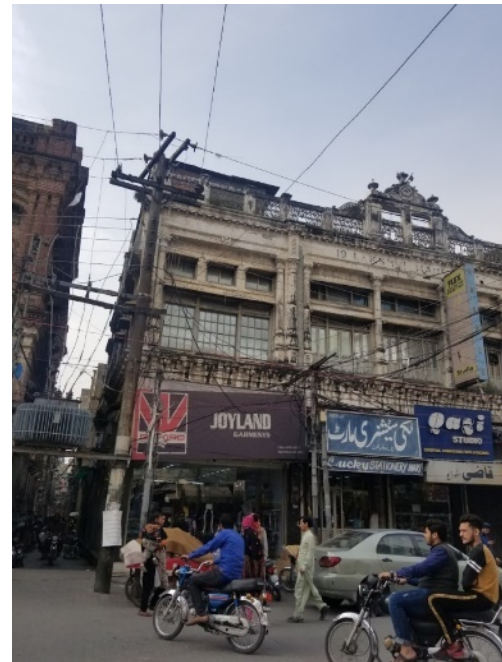
Figure 5. Offset from the adjacent building, Source: Authors (2022)
