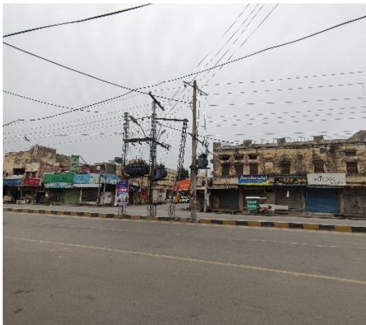
Figure 8. Poles were plastered with smooth cement, Source: Authors (2022)
