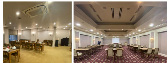
Figure 8. Air conditioners used in the hotel's restaurant and seminar room (created by the authors)
