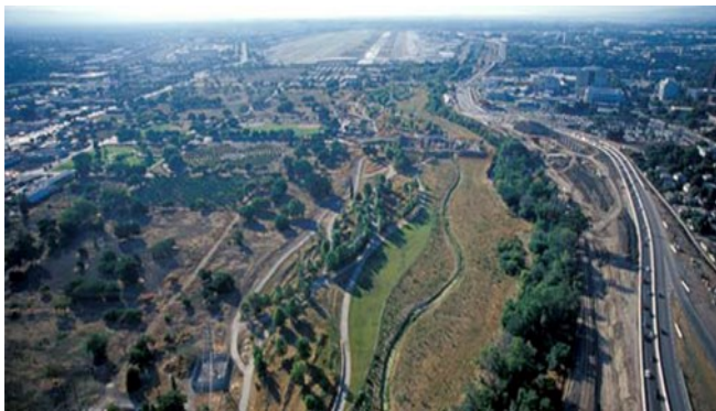
Figure 10: Guadalupe River Bank, San Jose, California, USA (Source: RIL, 2011)
