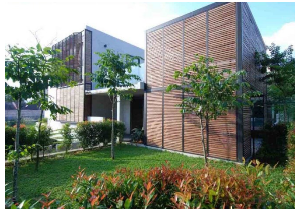
Figure 7: Denai House (Source: http://archinhome.com/wp-content/uploads/2009/09/ )
