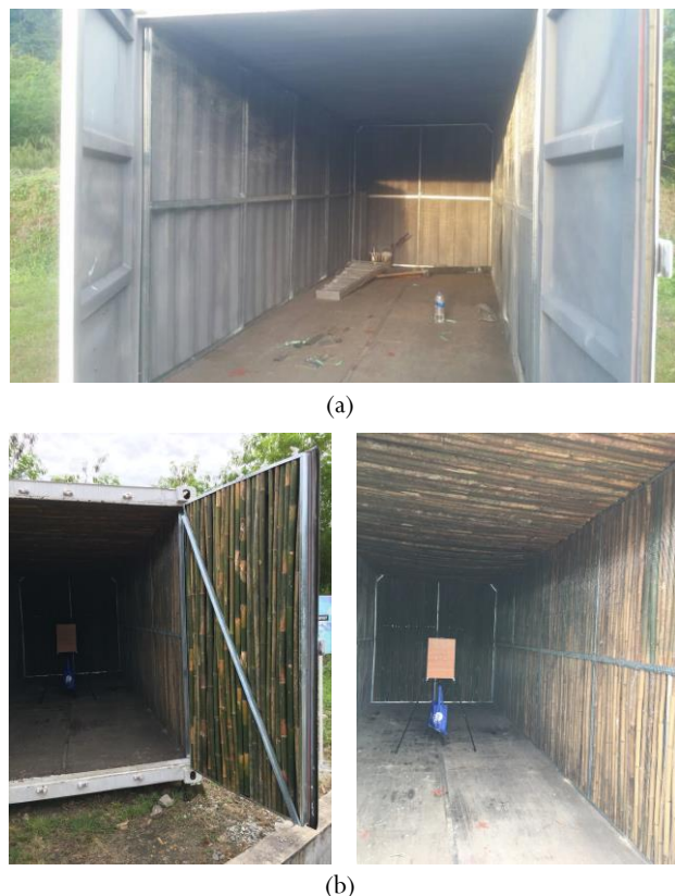
Figure 2 The arrangement of (a) bare unit of shipping container – BUSC, (b) shipping container installed with untreated bamboo as insulation – IUBSC
