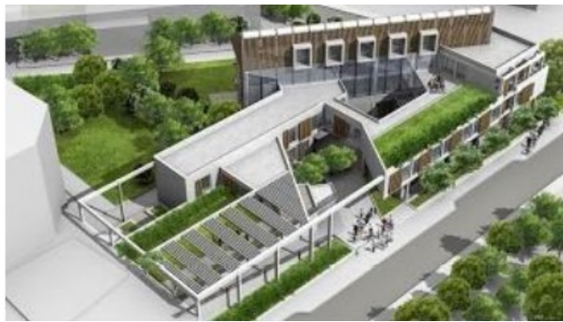
Figure 8 New Central Lecture Halls and Education Faculty buildings (TASAR, 2018)
