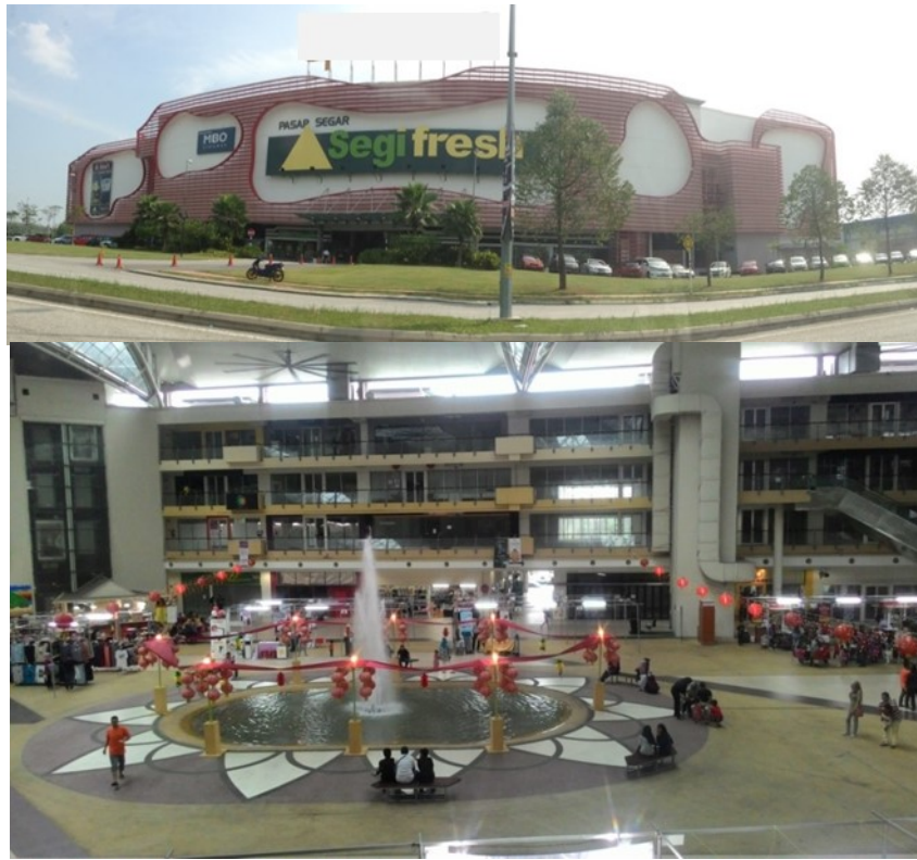
Figure 4: Exterior (above) and interior views (below) of SM2.
