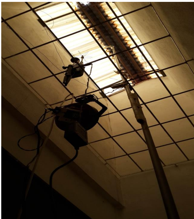
Figure 2 (a) and (b). The section drawing of the air well and test room in case study house. The (●) represents the position of the measuring point of HOB0 U12 air temperature and relative humidity data logger, which is 1.5m from floor level while (x) represents the HD32.3 Delta Ohm measurement logger placed 4.5m from floor. The photograph shows the location of C (Source: Author)
