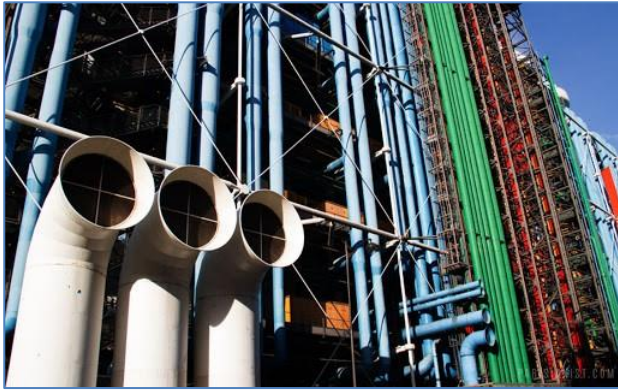
Figure 6 The Centre Pompidou to represent water (green), electricity (yellow), air circulation (blue) and people (red)
