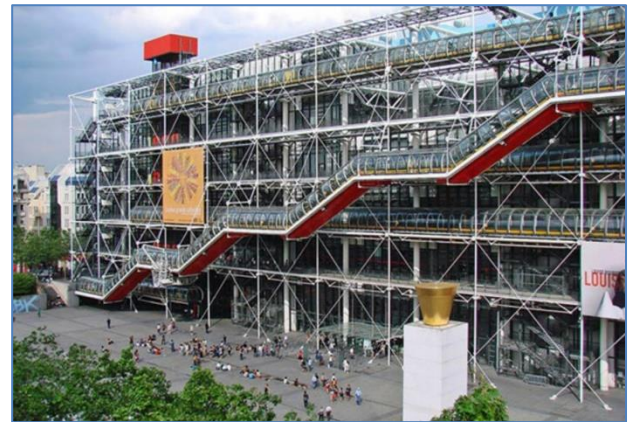
Figure 5 Exposed façade of The Pompidou Centre in Paris, with its elevator and interior design turned out
