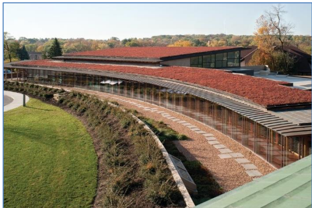
Figure 7: First Unitarian Society Meeting House with green roof design by Wright
