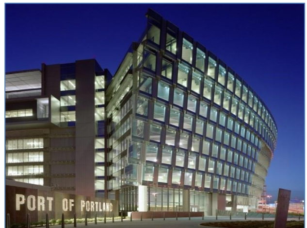
Figure 3 The Port of Portland headquarters, inspired by the hull of a ship
