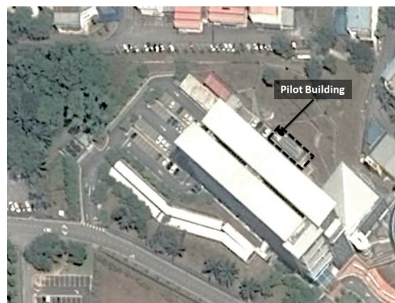
Figure 11 Aerial view of the building site
