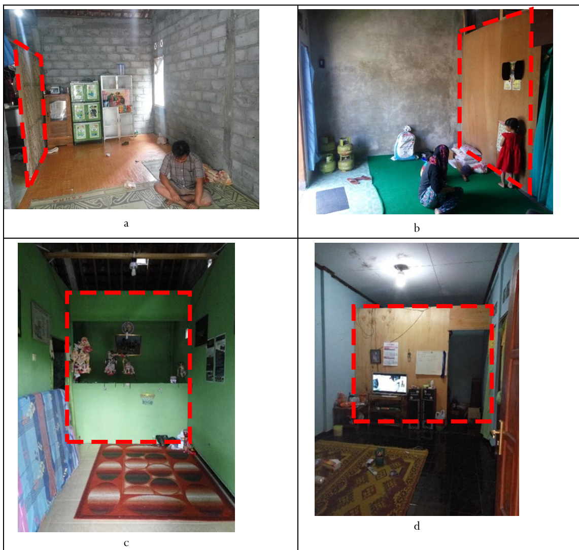
Figure 6. Architectural elements as the space divider in Pagerjuran permanent shelter (Author)
