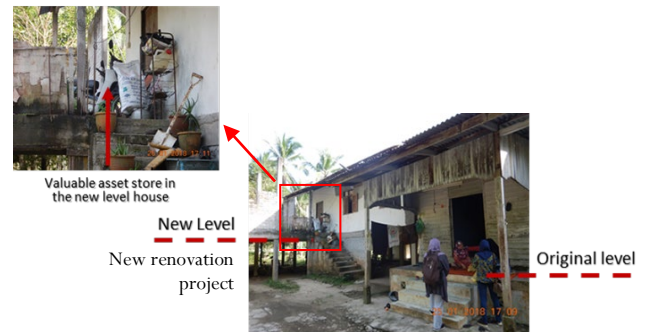
Figure 7 (from left) Valuable asset store in the new; (right) House elevation is raised to a new level to surpass the highest flood water level recorded over the years
