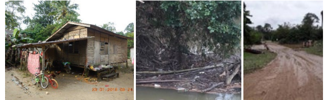
Figure 4 Physical damages caused by flooding. (Photo, from left) wooden house structure damage by flood, debris in the river and main road in the village was covered by thick mud after flood receded
