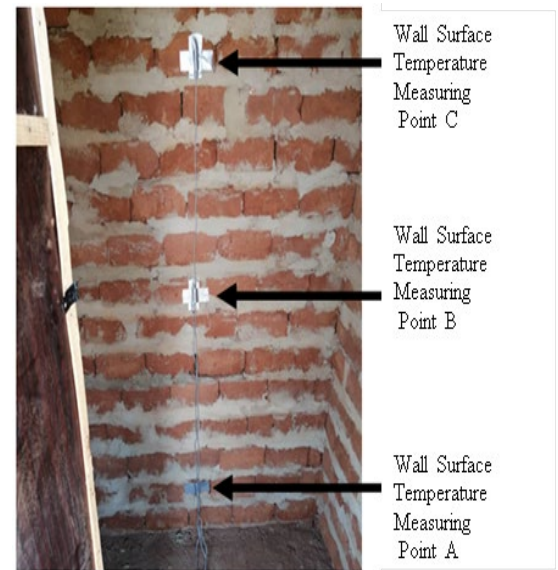
Figure 9. Internal Walls surface temperature measuring points
